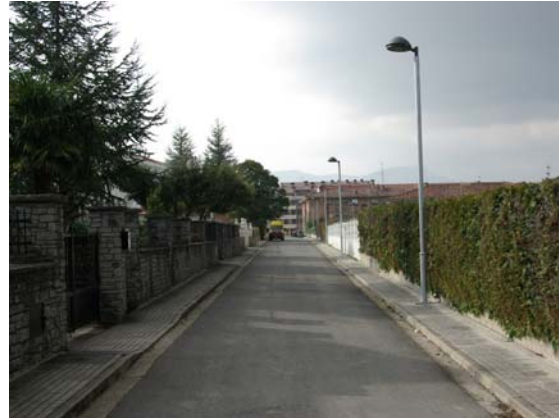
Calle renovada, luminarias FHS_{inst} = 0\%
