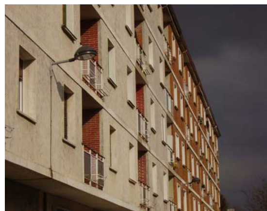
Calle renovada, luminarias FHS_{inst} = 0\%
